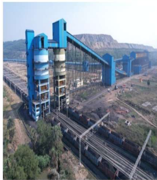
CHP (10 Mt) Built at Sattupally, Telangana
